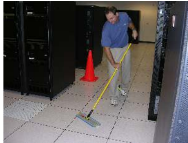
Raised Floor Cleaning
